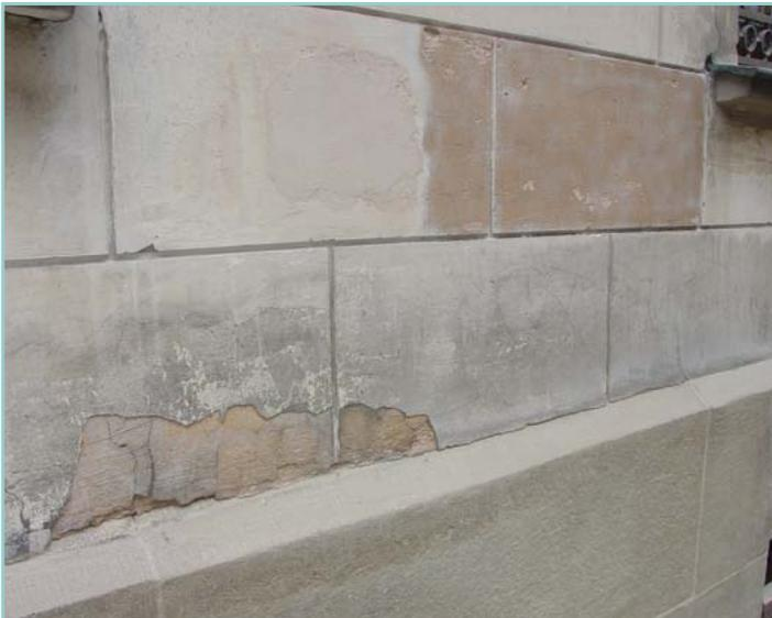
Cleaning has revealed the original surface of the render.
