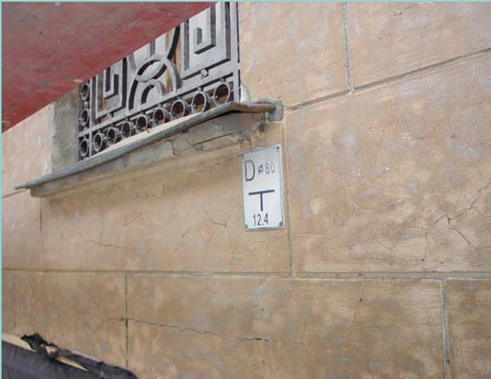
After the removal of the secondary cement coat, changes in the original appearance of the renders became visible: stains due to salts and soiling and dirt penetrating the network of cracks.
