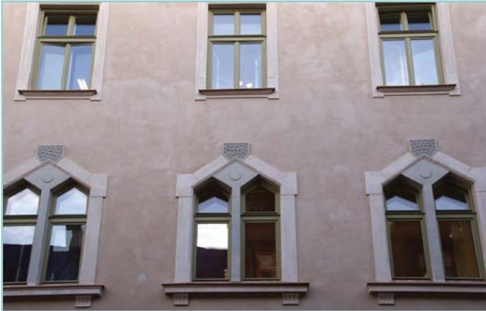
The renders were re-integrated aesthetically with a thin layer of Roman cement mortar and coated with the water repellent silicone paint based on Roman cements, both produced by the Institute of Ceramics and Building Materials, Branch of Glass and Building Materials in Krakow, Poland.
